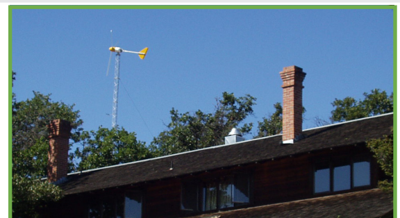
A properly designed wind turbine installed above surrounding obstructions
